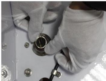
**Step 7:** Screw the retaining nuts tightly on to the reactor chamber. Starting with the bottom nut first and then the top nut.
